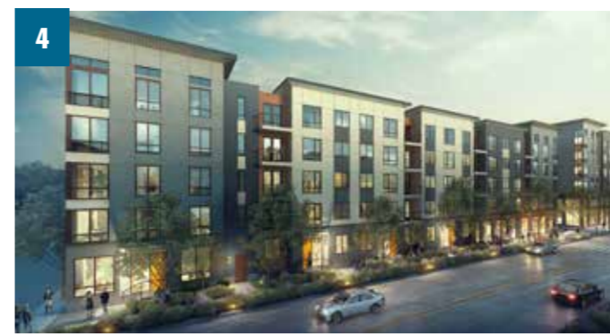
4 Alvarado-Antonio Apartments 899 Alvarado St. • 5.73 acre Transit Oriented Development • 687 residential units mix of studios, 1, 2, and 3 bedrooms
